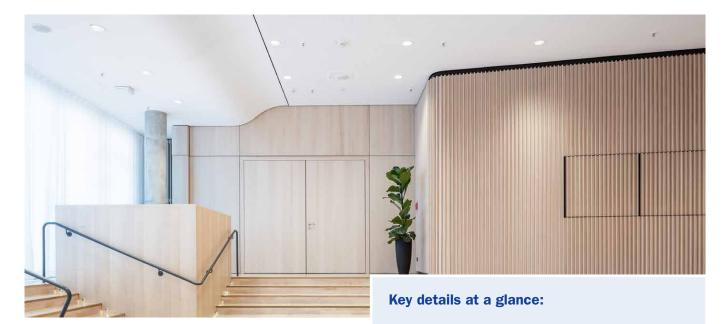
This project was executed using dimensionally stable modules made of steel frames, chosen in part to meet fire protection requirements. These modules were pre-fitted at the factory with brackets for lighting fixtures and notches for CD profiles and the on-site curtain rail. The components were installed around the girders using installation templates, and the varying linear sections between the girders were then connected with CD profiles.
